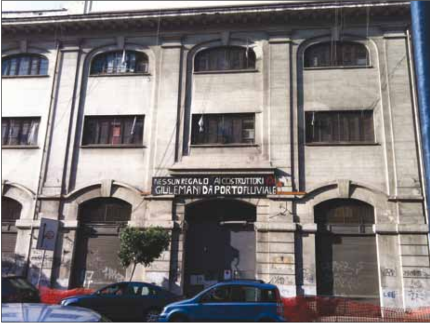
Figure 10 Porto Fluviale: the outside, 2012. Photo: DPU summerLab.
