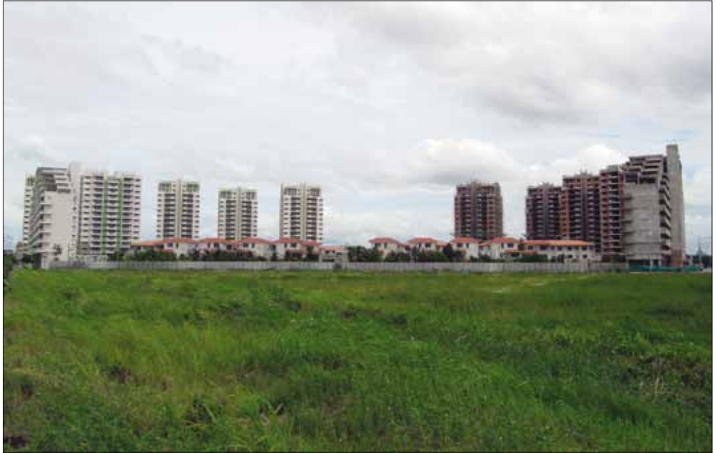
Figure 1 CamKo City under construction. Photo: Giorgio Talocci.
