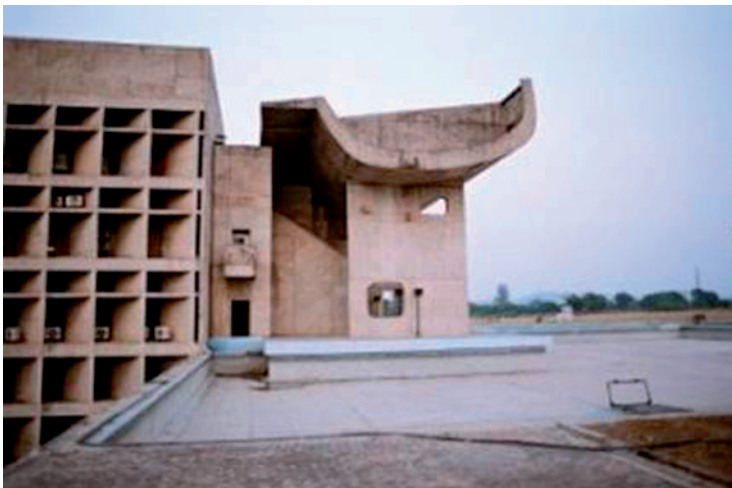
Secretariat, Chandigarh, photo taken in 2006 by Danny Hanlon ( http://dannyhanlon.com/blog/2006/12/20/chandigarh )
